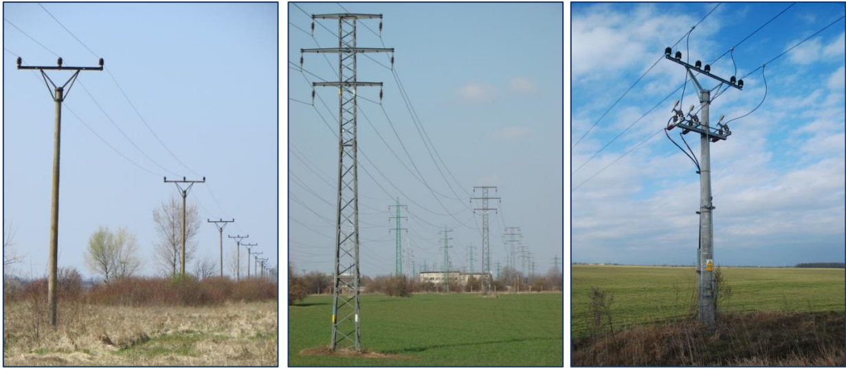
Utility poles of 22 kV line in Slovakia
