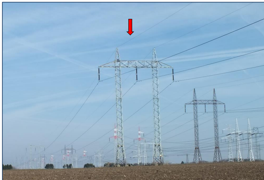
Fig. 23 The thinnest (shield) wire on the top of the power lines is almost invisible for birds
