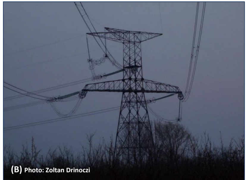
Pylons of 2x400 kV power lines in Hungary (A) and 750 kV in Hungary and in Ukraine (B)
