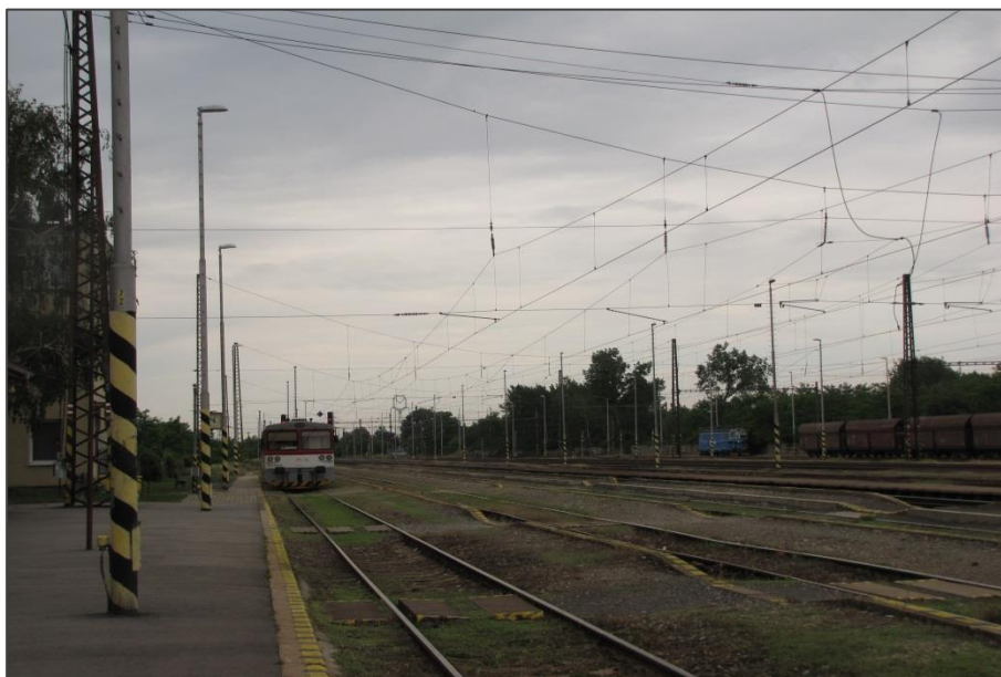
Fig. 5 Electric railway power lines
