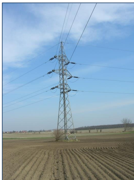
Pylons of 2x110 kV lines in Slovakia
